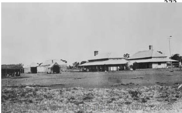
373 Figure 9. The Tennant Creek Telegraph station in 1872, showing a wind vane and Stevenson screen on the far right of the photograph (National Archives of Australia Item ID: 11774998). As the site was close to buildings, it was probably watered by bucket or watering-can during the seasonal 'dry'.
