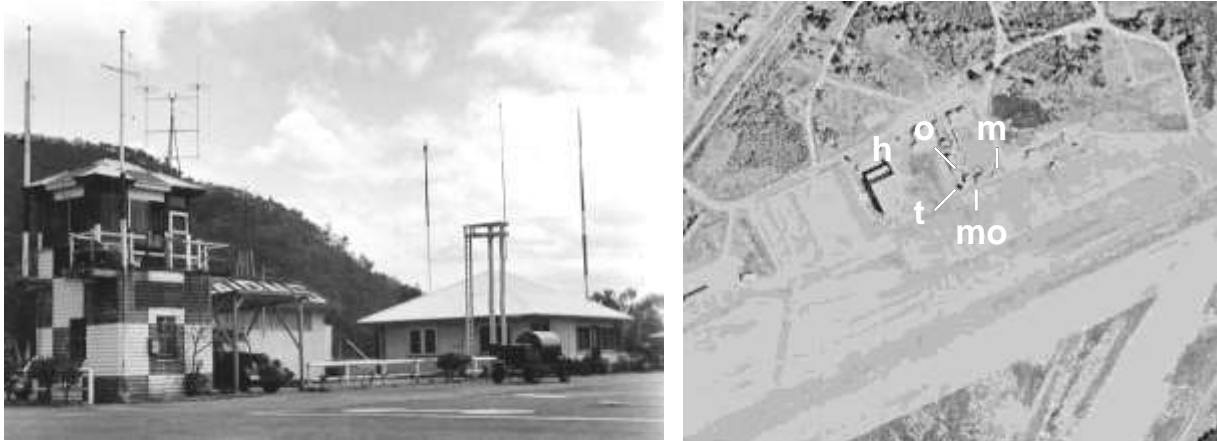
Figure 1. Cairns control tower, operations centre (behind) and the Aeradio met-office in c. 1959 (left). The 40-foot (12m) anemometer and windvane (usually mounted on the roof) charted windspeed, duration and wind direction. The signal square in front of the control tower was used for emergency visual communication with aircraft. Radio operators originally occupied one side of the 1940s Aeradio office and met-staff the other and a vestibule was used for pre-flight briefings. In 1946 post-WWII functions were split between the Department of Civil Aviation, which later became Flight Services (responsible for air-traffic control) and the Weather Bureau, which became the Bureau of Meteorology. (Photographed from airside courtesy of the Civil Aviation History Society (CAHS)). An airside view of the operating precinct in 1952 (right) shows the main hanger (h), control tower (t), operations centre (o), met-office (mo) and met-enclosure (m) (portion of QAP0298012 1 ; 30 June 1952).
